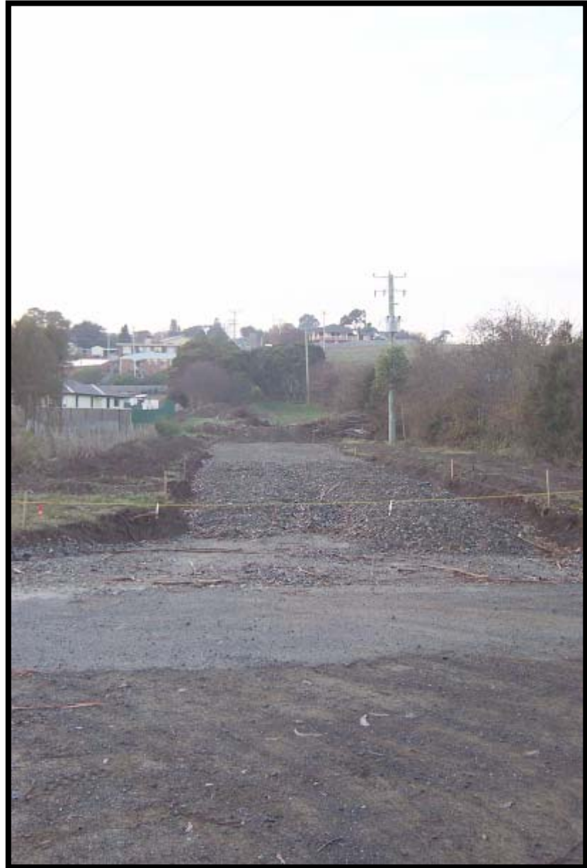
Road Continuation through Trevor Street
